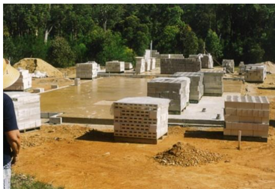
The donated blocks ready for laying
