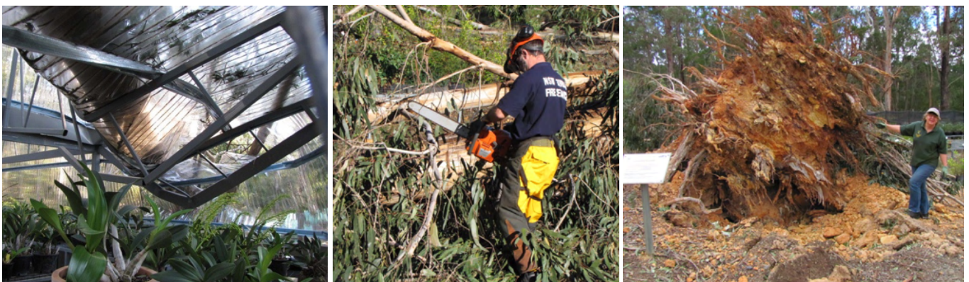
Orchid House destruction after windstorm, NSW Fire Service helping with clean up, tree down on site.
