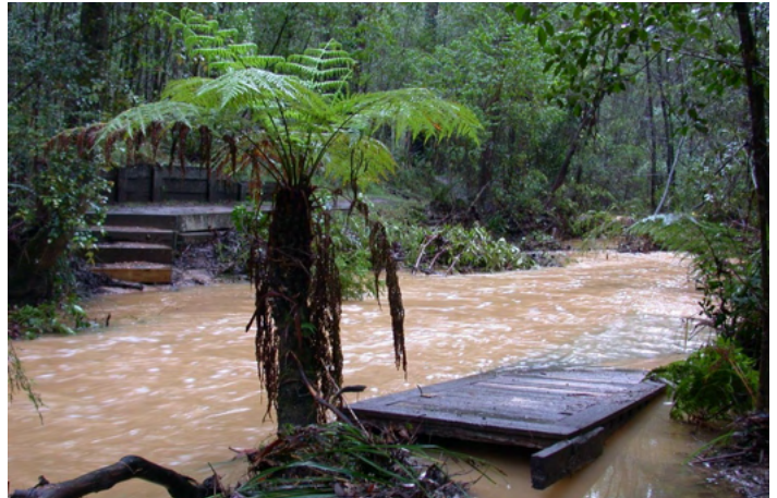
Bridge on track 3 is washed away, 2007
